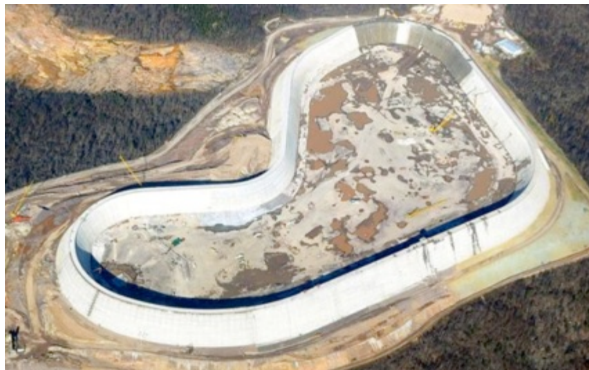
Figure 30: Taum Sauk PHES dam under reconstruction with roller-compacted concrete. (KTrimble, 2009)
