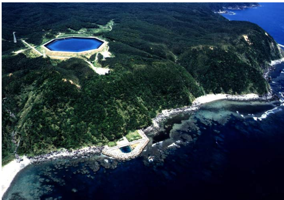
Figure 12: Yanbaru seawater PHES plant on Okinawa Island, Japan. (Renew Economy, 2013)
